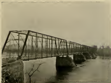
CONNECTICUT RIVER BRIDGE
